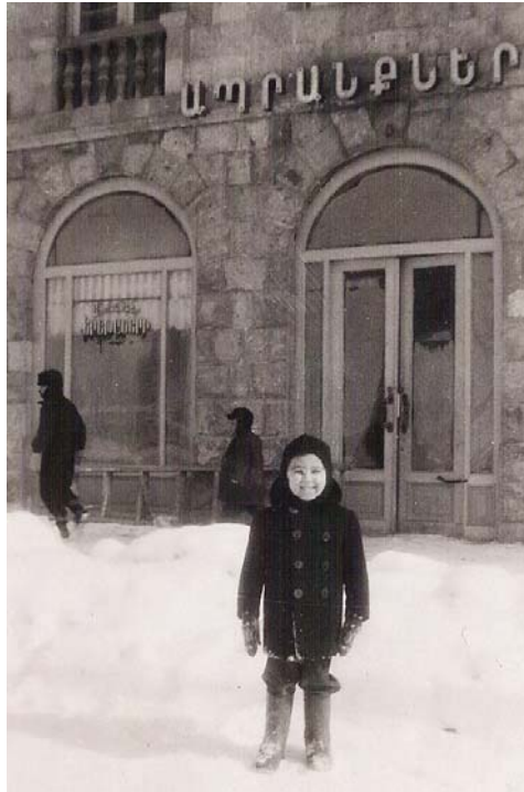
Diran, residential block and provision store, 1950.
